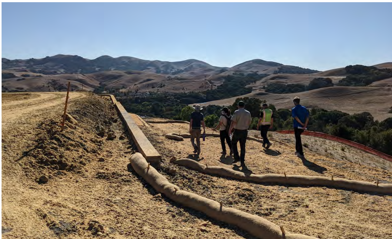
The Saudade Walk-in Entrance from the Faria Preserve HOA area will connect trail users to the Calaveras Ridge Trail (seen under construction in the photo above).
