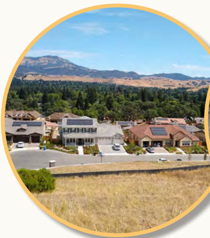
4. View of Wingfield Court from Podva property
