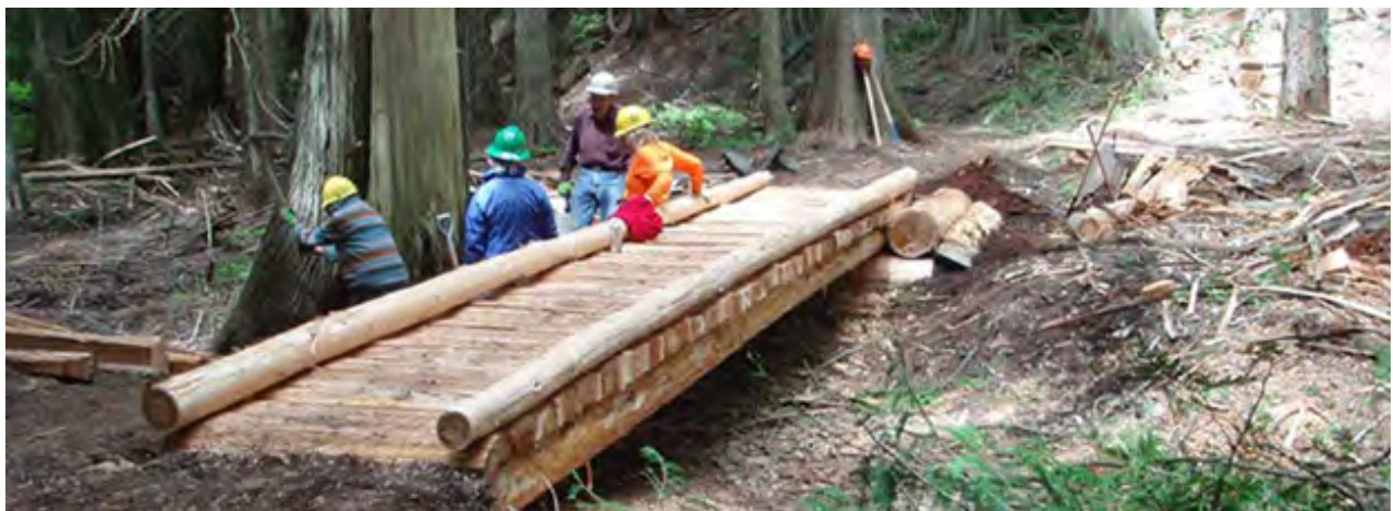
Puncheon structure constructed by the NE Chapter Back Country Horsemen of Washington
