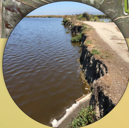
2 Repair Eroding Levees
