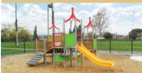
Playground Installation, Concord
